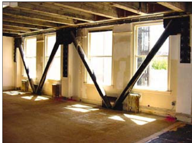
Steel bracing was used in areas such as window walls.
